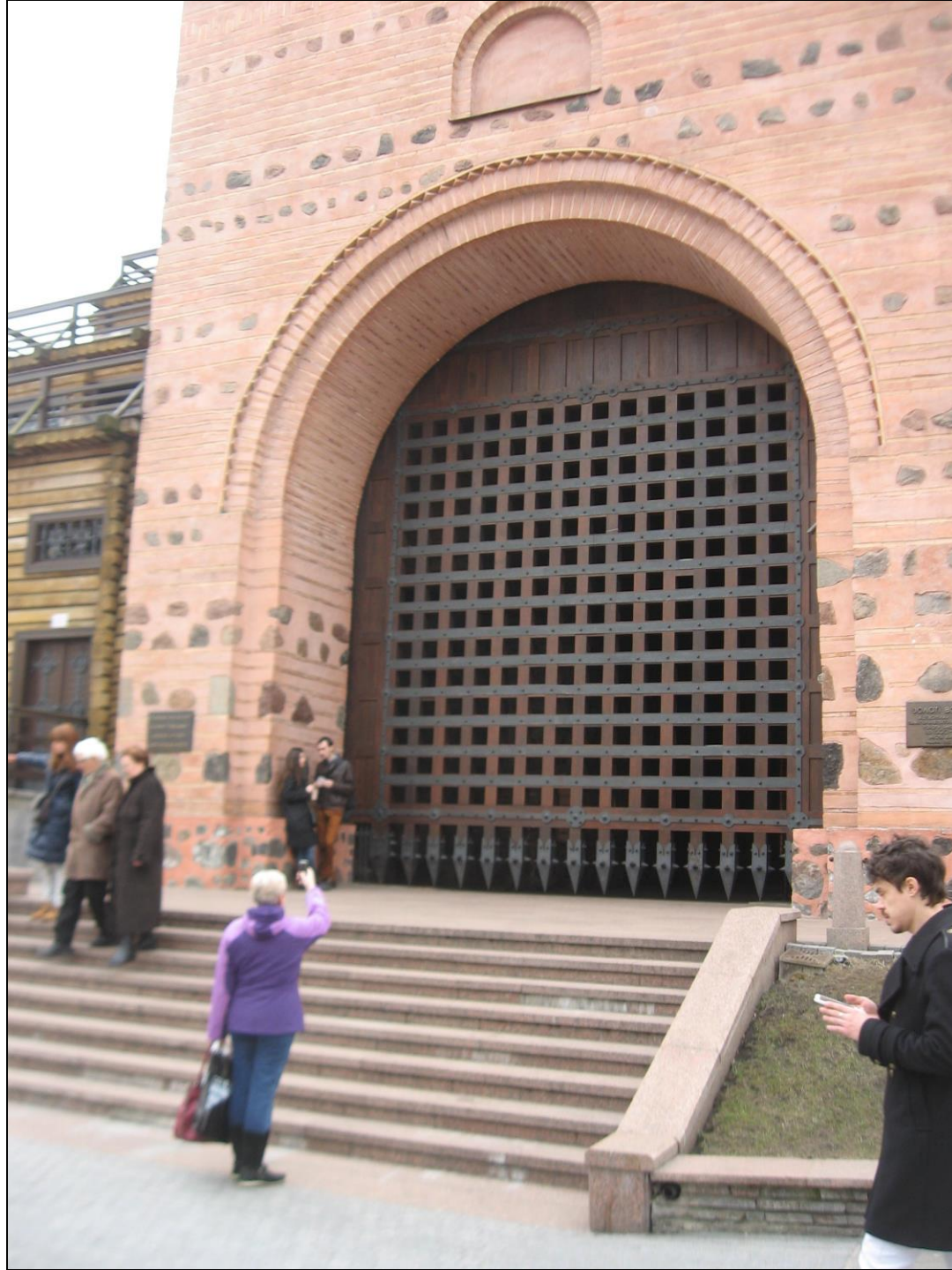
Golden Gate at backside of St. Sofia
